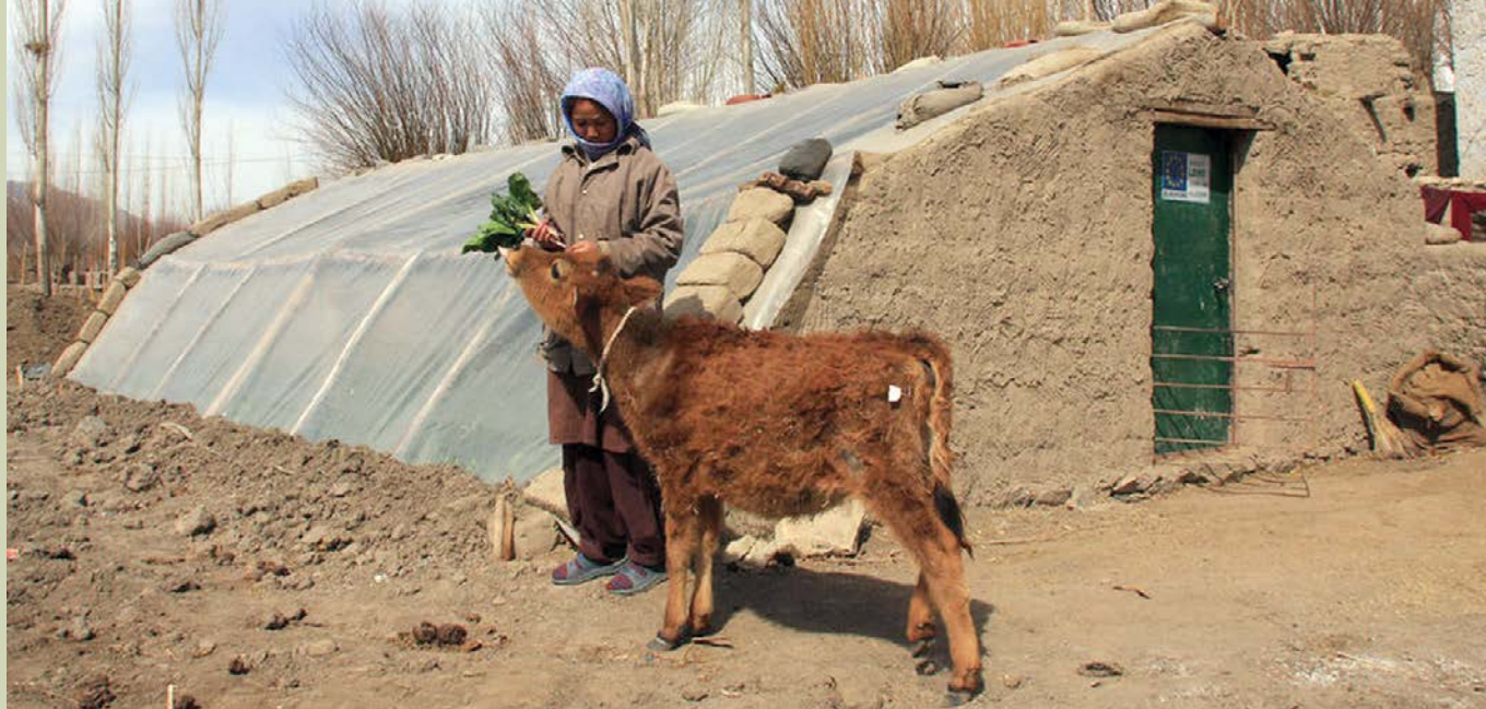
Solar Greenhouse in Ladakh, India. Designed to trap and store the sun's heat to grow food during the winter
